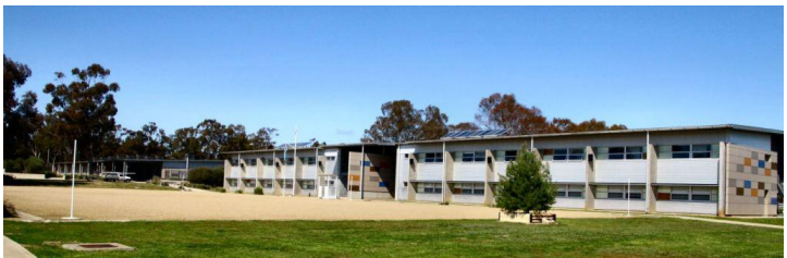
Figure 1: 1RTU Living in Accommodation
